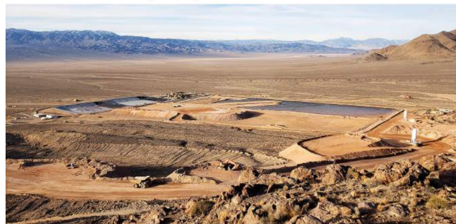
Overlooking Heap Leach & Process Facilities
