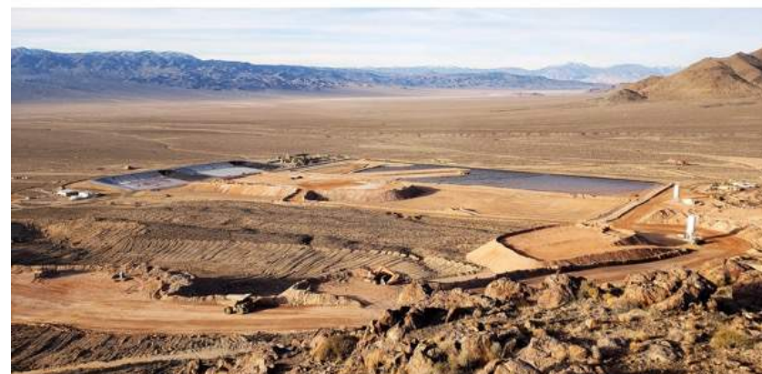
Overlooking Heap Leach & Process Facilities
