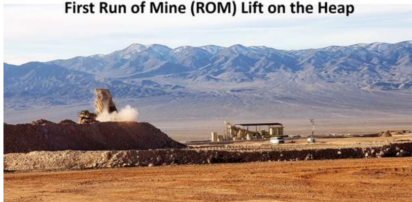
Overlooking Heap Leach Process Facilities First Run of Mine (ROM) Lift on the Heap
